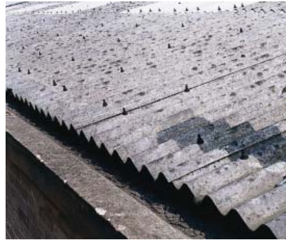
Asbestos cement roof tiles
